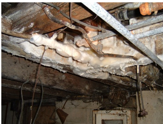
Figure 2. Frozen plumbing and mold growth on floor joists. Note, some of the mold growth is white.
